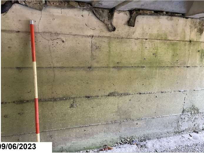
Bent 2: couple of vertical cracks in the abutment near mid span
